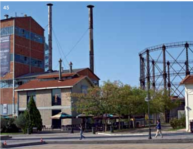
44. Part of the old Gasworks facility was turned into an Industrial Gas Museum.
